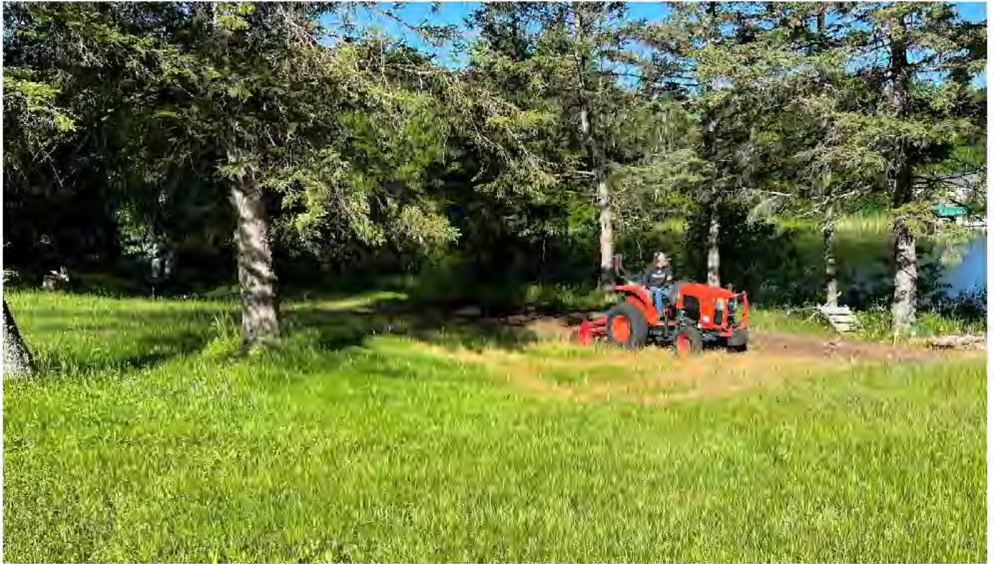
Beginning Stages of Construction - Contractor using a Harley Rake to break up the hard-compacted soil present at site.
