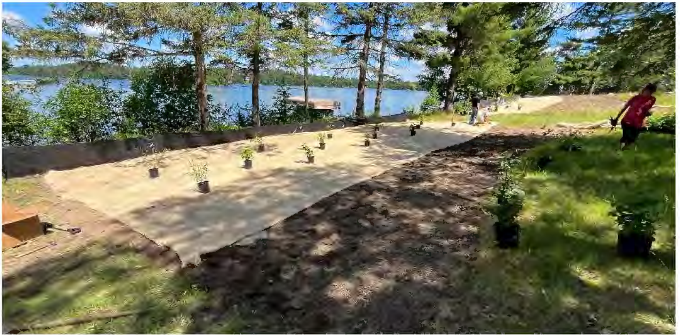
Middle Stages of Construction - Contractor in process of laying out erosion control blanket and staking it in.
