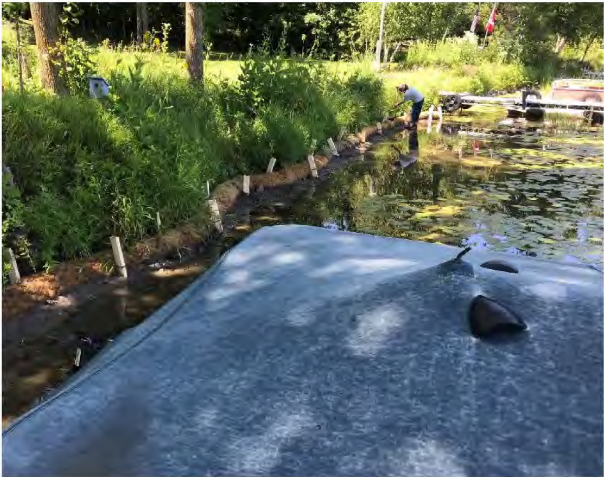
Coir Log after install
