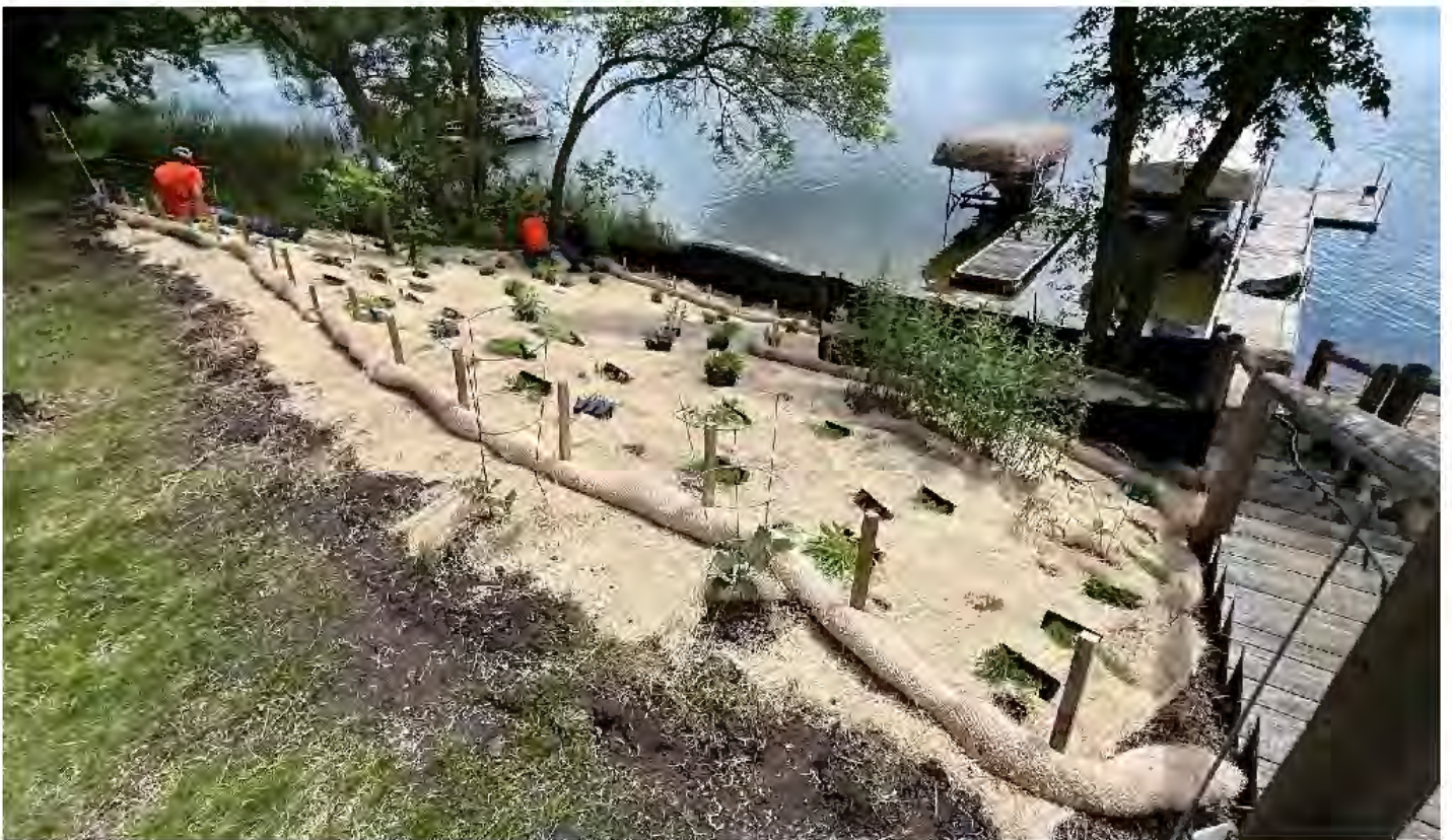
Final Stages of Construction - Contractor planting native plant plugs
