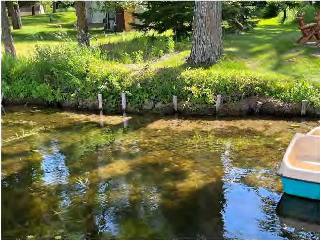
Coir Log After Repair
