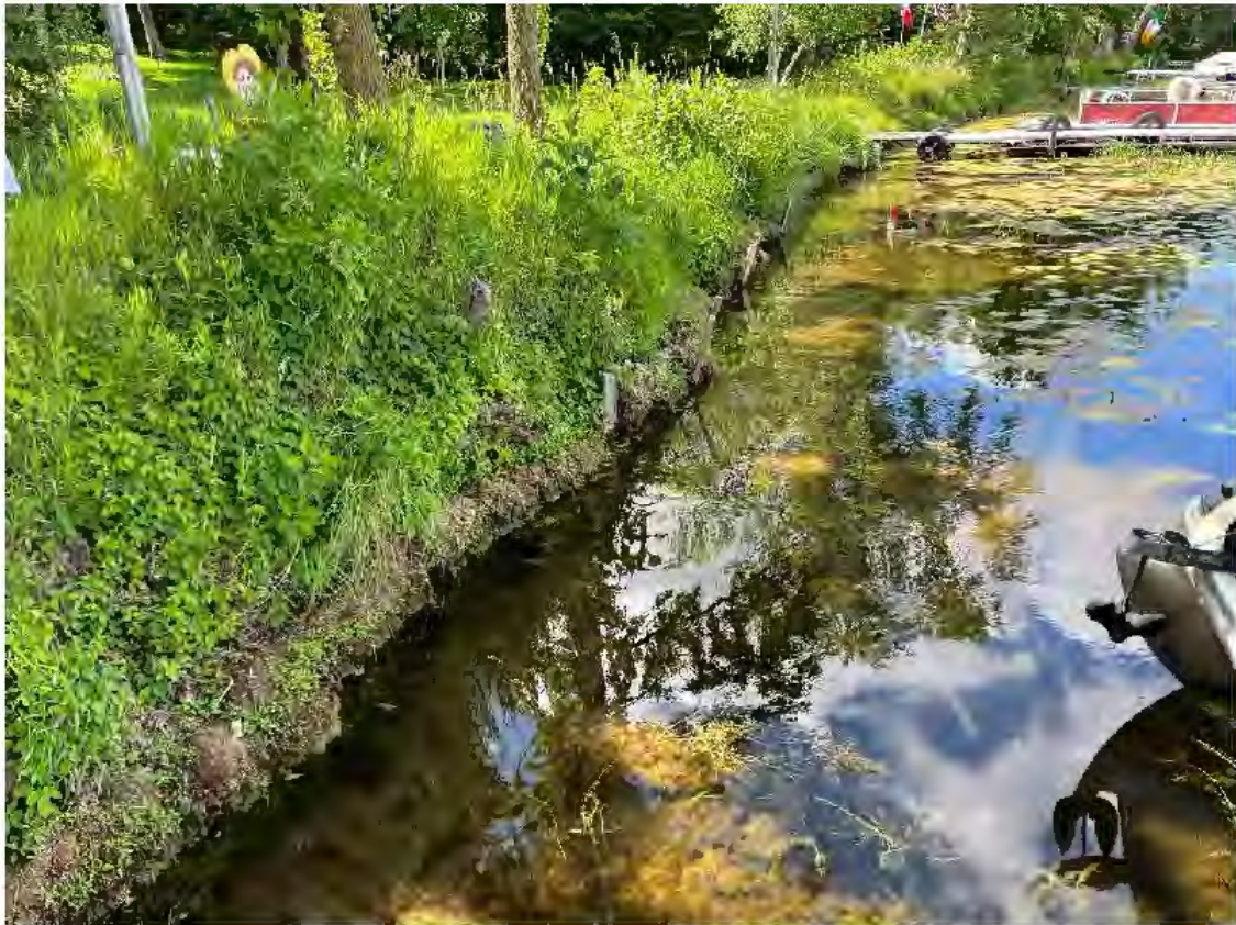
Coir Log After Repair
