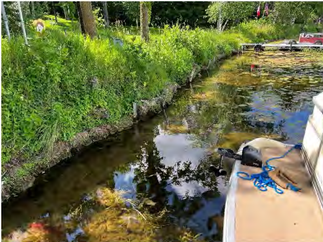
Coir Log After Repair
