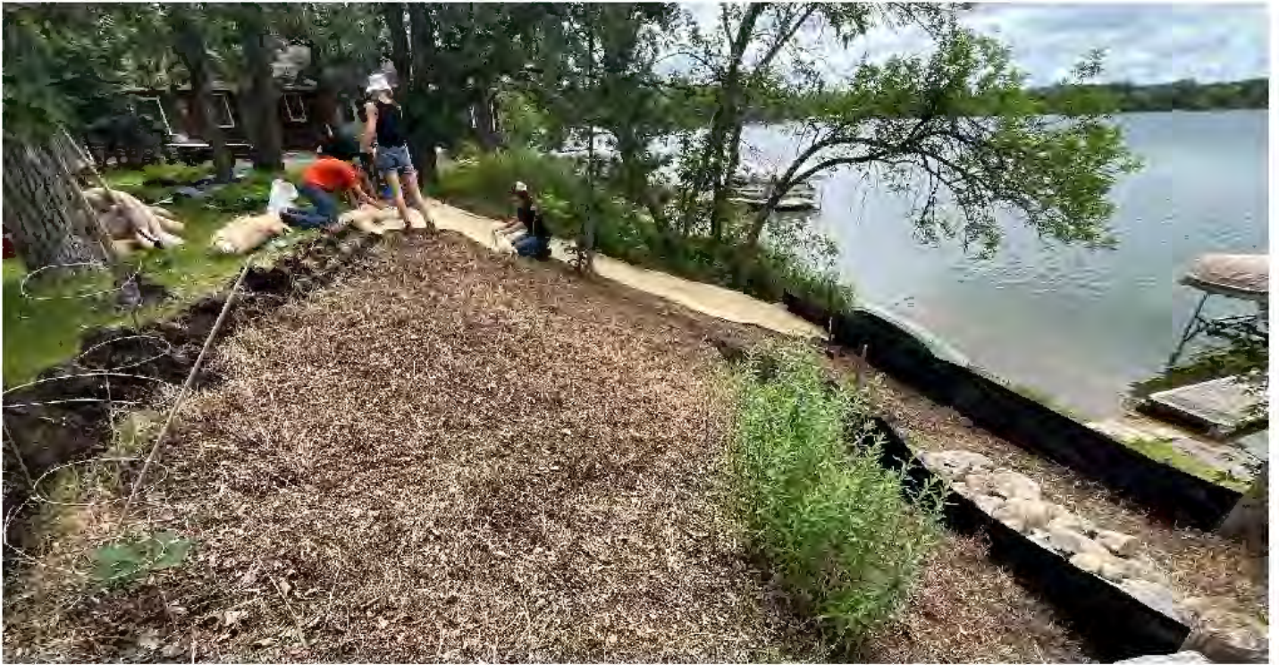
Middle Stages of Construction – Contractor Laying out erosion control fabric over seeded area
