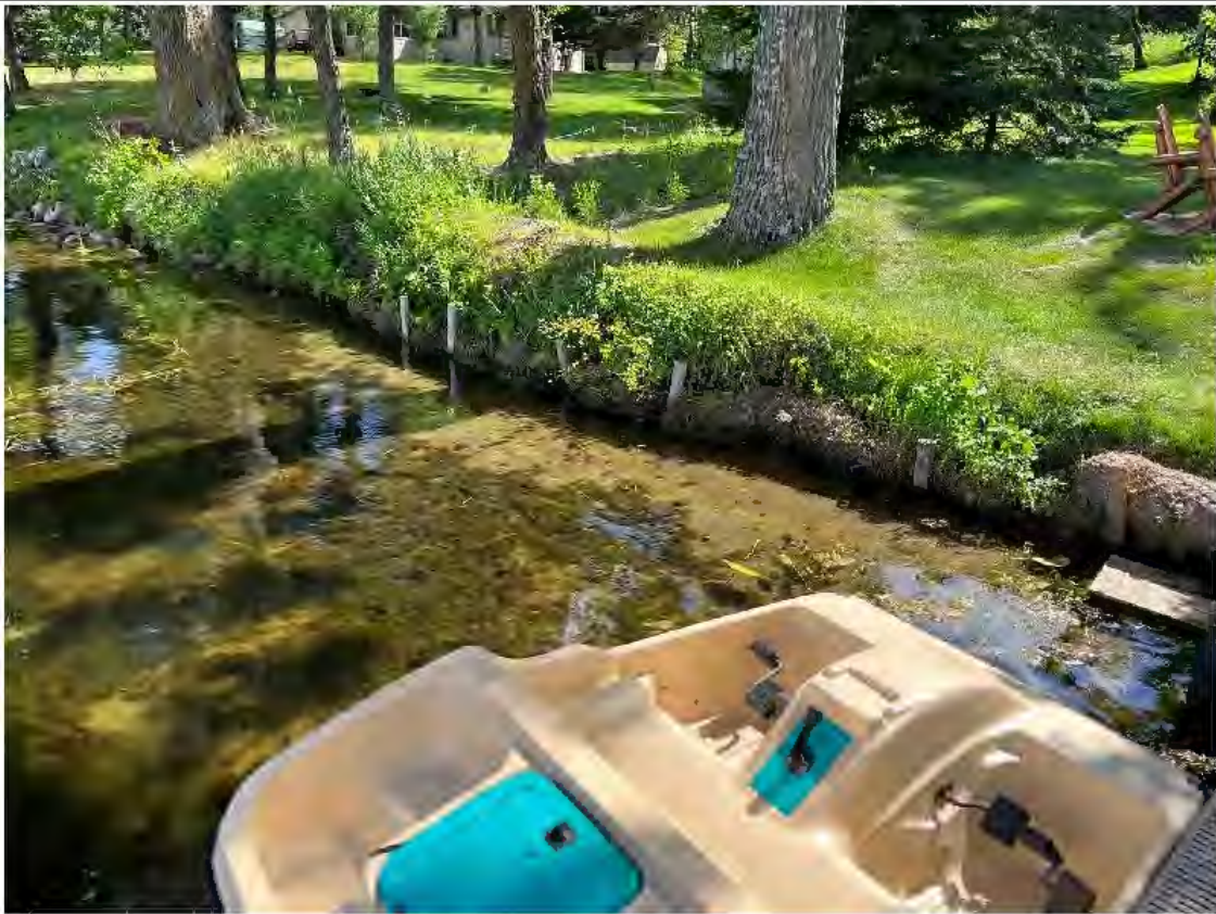
Coir Log After Repair
