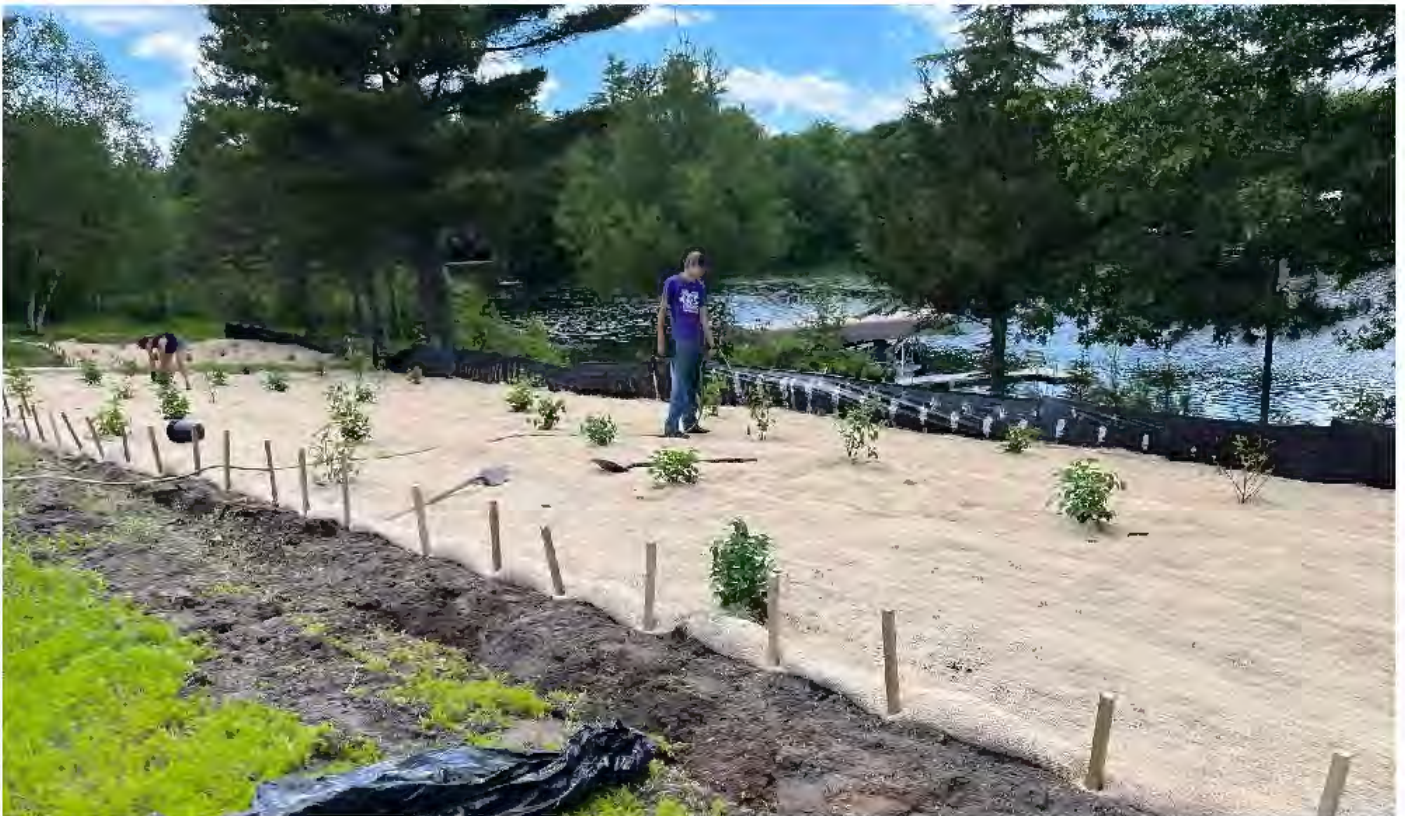
End stages of Construction - Contractor in process of planting the shrubs.
