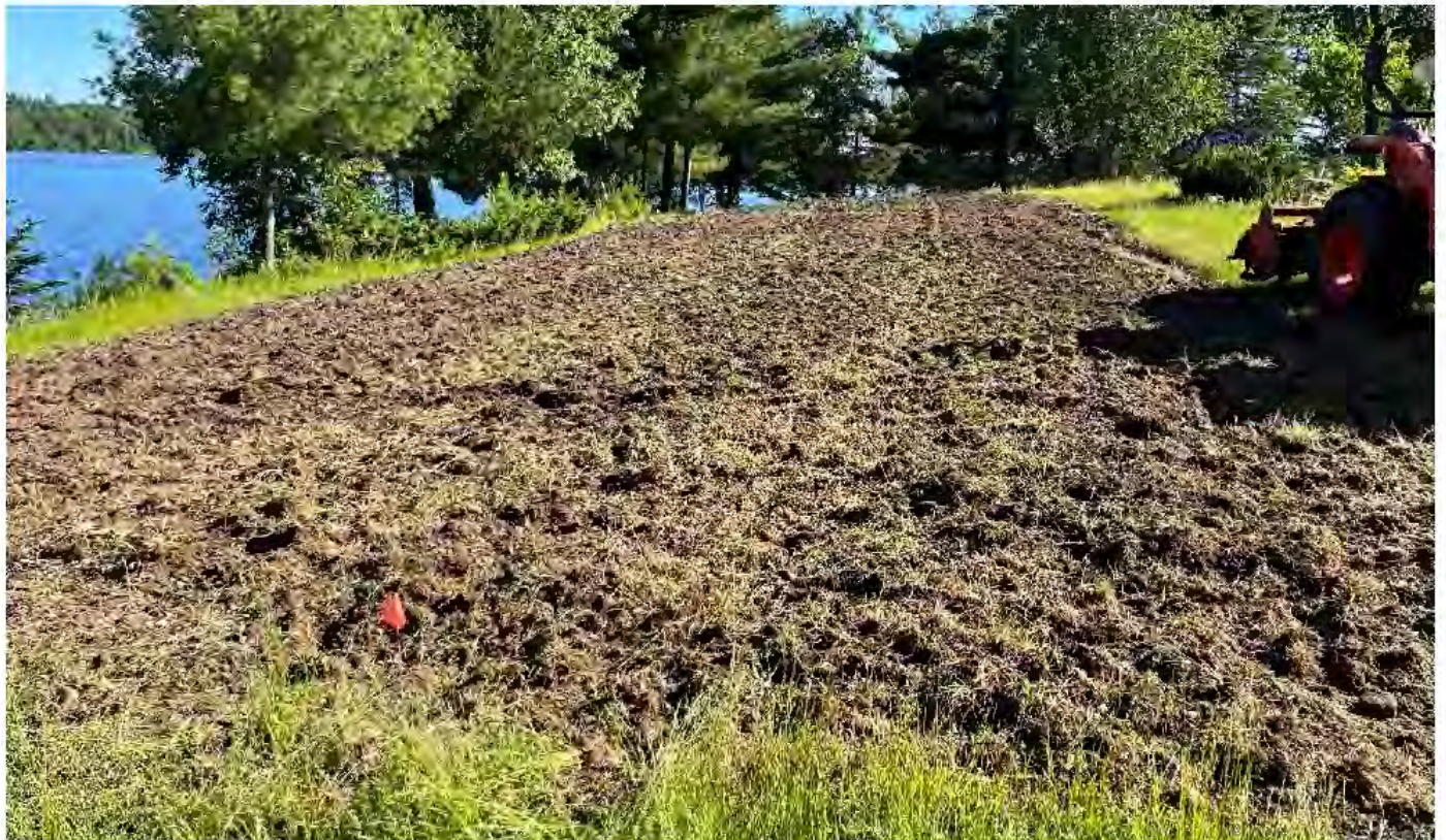
Beginning Stages of Construction - Contractor using a Harley Rake to break up the hard-compacted soil present at site.
