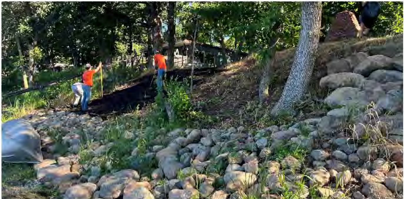
Early Stages of Construction - Topsoil/black dirt brought in for eroded areas of bank
