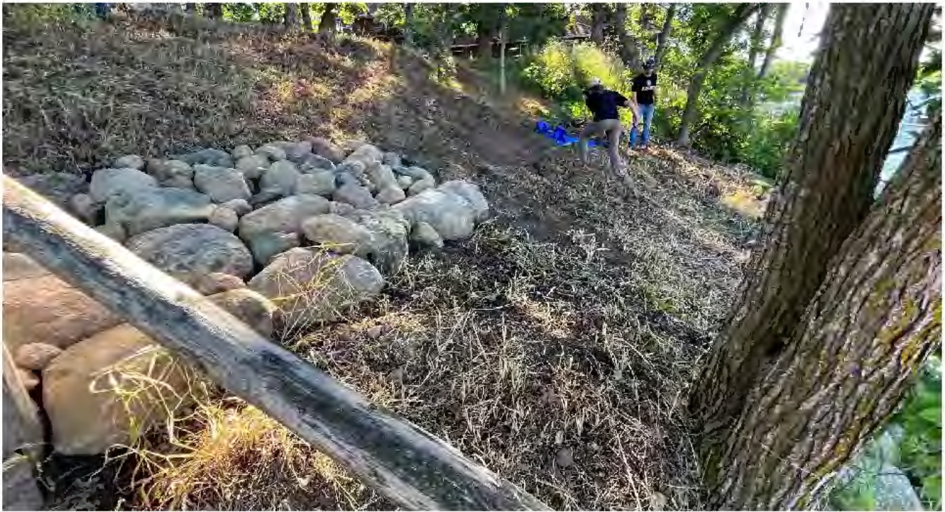
Early Stages of Construction – Contractor removing existing vegetation and creating seedbed for native seed mix.
